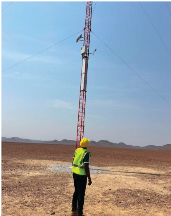
Above: MET Masts have been set up on site to record wind data at a height of 130 meters
